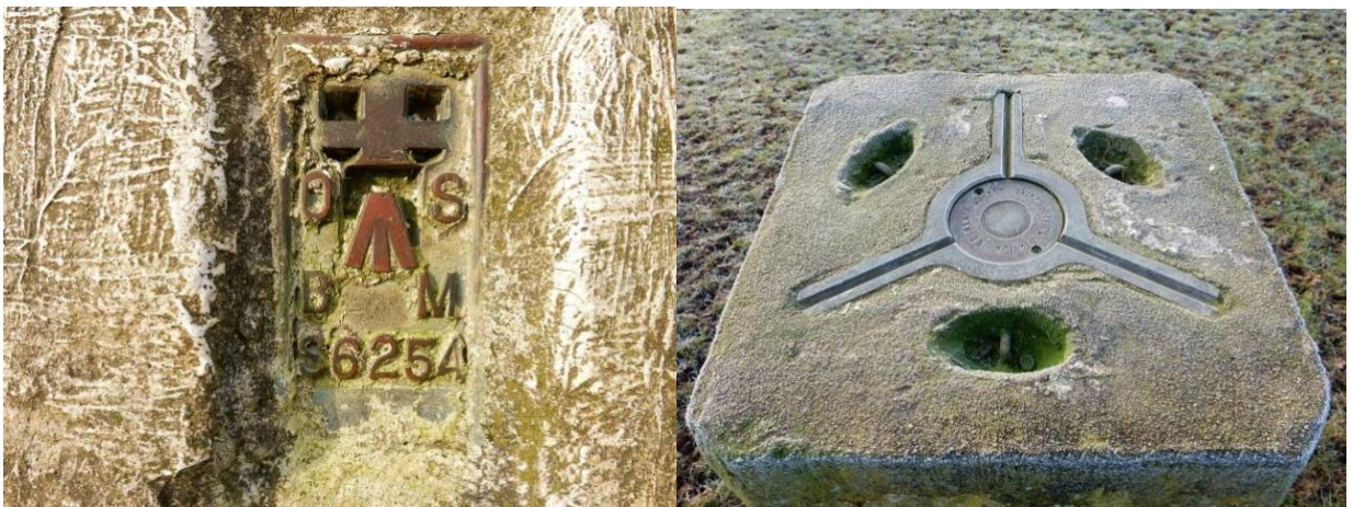
Photo: Trigonometry Point on Plaistow Mount, Nell Ball Hill, Plaistow (2006: left: flush bracket; right: pillar top).
